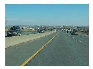
This is a picture I took showing how low the center concrete barrier is along this stretch of highway. The low height allows drivers to easily see the headlights of oncoming traffic at night.
